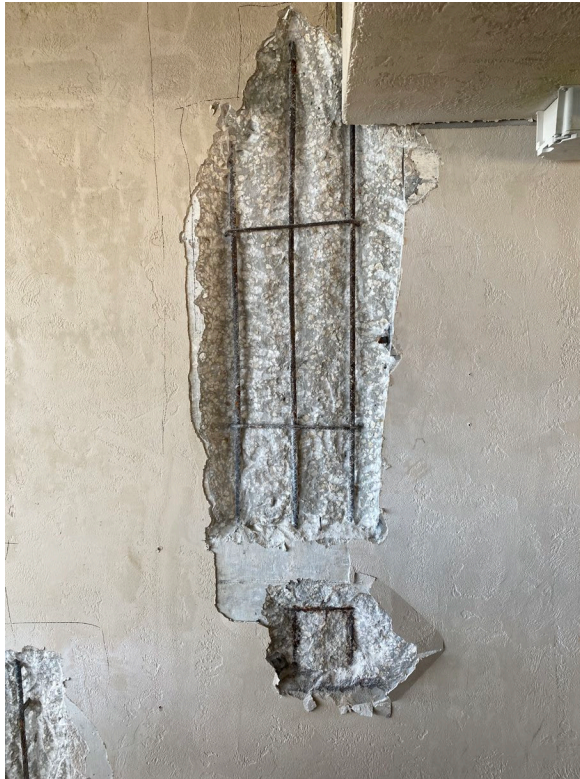
Picture 4: In-progress demolition in garage
