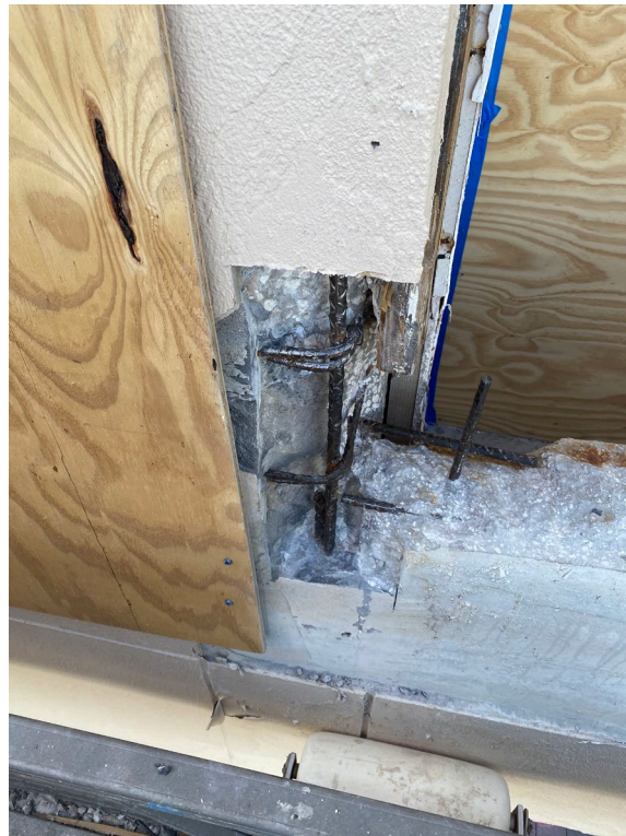
Picture 2: In-progress repair at Unit 110 prior to steel supplementation
