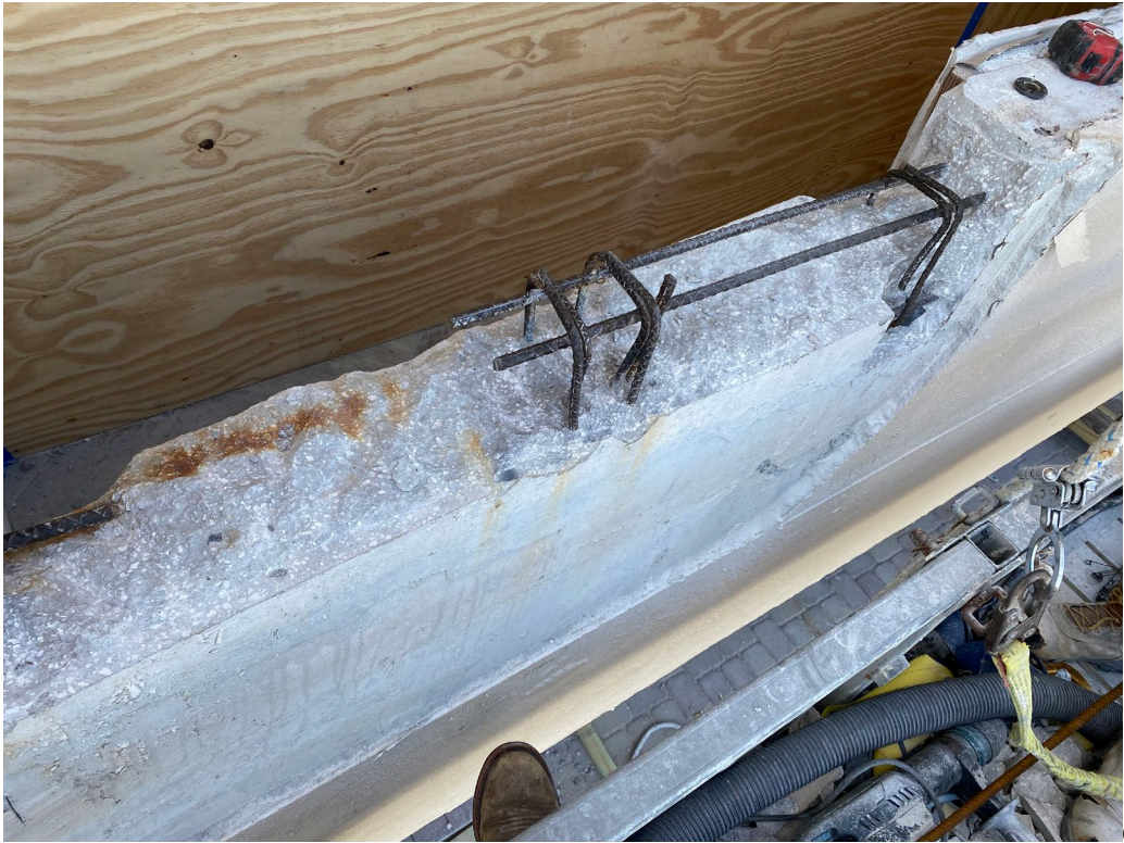
Picture 1: In-progress repair at Unit 110 prior to steel supplementation
